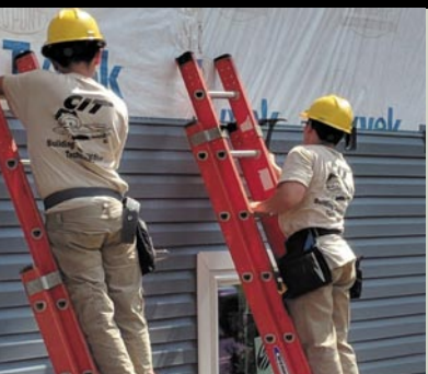
Building Construction students complete the siding on the house.
