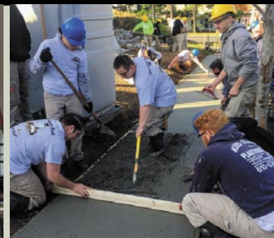
Masonry students lay the concrete for the sidewalk
