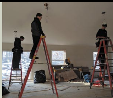
Electrical Construction students install recessed lighting in great room.
