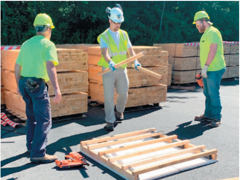
Center - Ben Page from Pa. Fish & Boat, shows Upper Mt. Bethel TWSP. Volunteers how to build a crib from a template.
