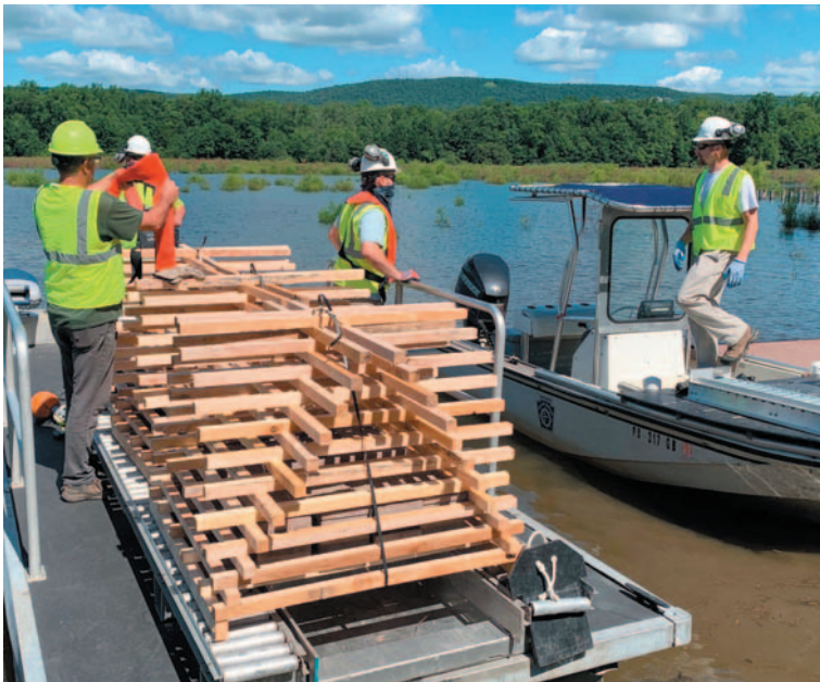
Porcupine cribs were loaded onto boats and driven to GPS locations on the lake and dumped in. You can find their locations on PA Fish & Boat website.
