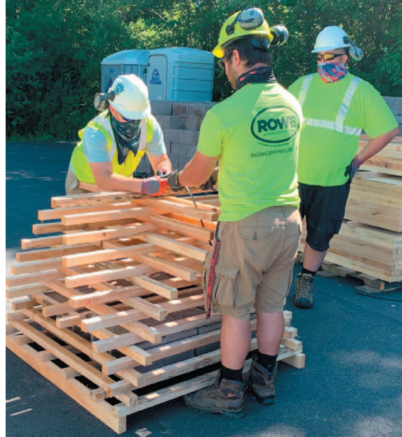
Center - Ben Page from Pa. Fish & Boat, shows Upper Mt. Bethel TWSP. Volunteers how to build a crib from a template.
