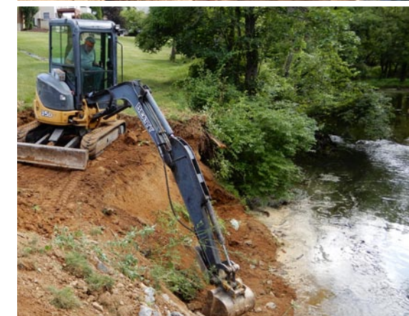
Contractors, volunteers and Northampton County Parks staff stabilizing & planting a steeply eroded streambank at Gertrude Fox Conservation Area last summer.
