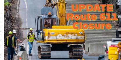
sections of concrete barriers. They are removing the sections, shoring up the base material for support, and then resetting the section. Once this is complete, four areas of the roadway must be repaired. Two areas will be shored up with fill material, and the other two will have concrete slabs constructed to provide support for the roadway.
