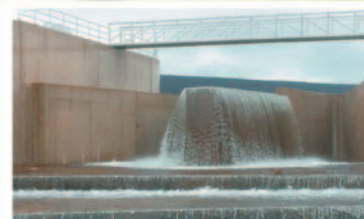
Install a pedestrian bridge over the new spillway
