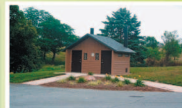
Construct new restroom facilities
