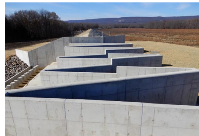
The completed dam
