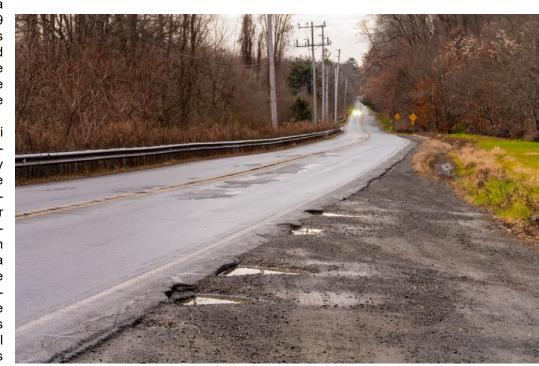
recreational facilities located along the corridor, however it is currently in very poor condition with failing pavement, poor drainage, and numerous potholes."
